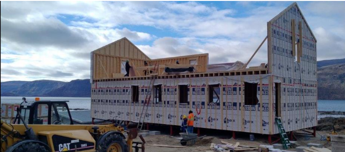
Pangnirtung office building under construction in September 2016
